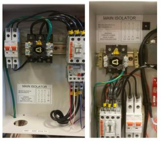
Figure 3-11, Main Isolator Wiring
