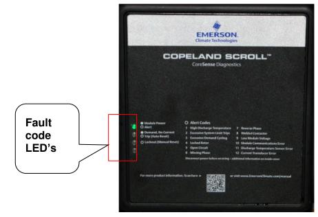
Figure 5-3, Emerson Compressor Front Panel Fault Code LED's
