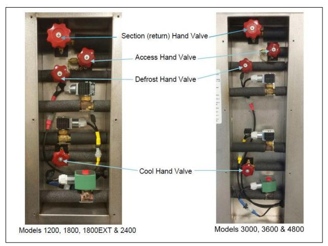
Figure 3-5, Position of Hand Valves
